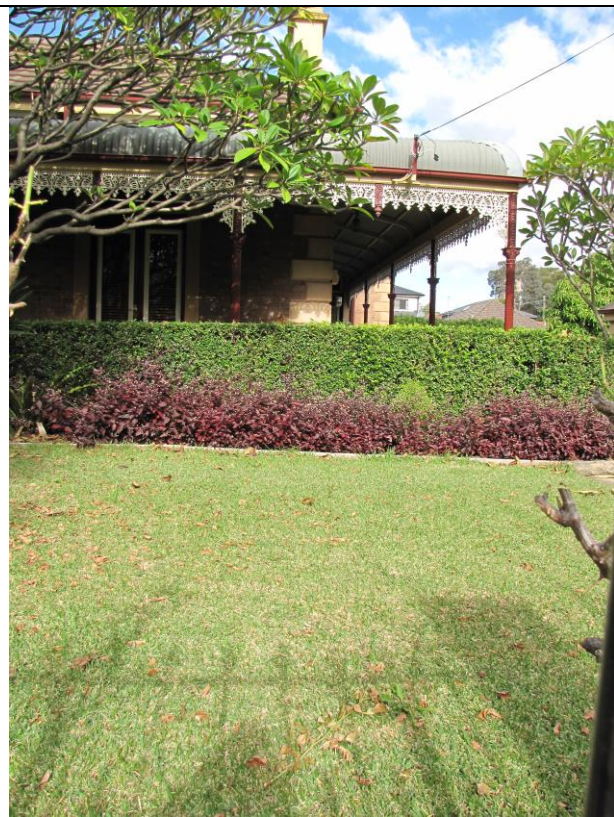
Front verandah - northern western corner.
