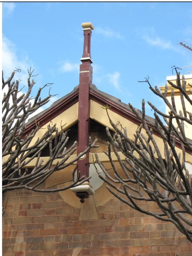
Detail projecting front bay, flying gable and finial, sandstone circular vent – sympathetic period colours.
